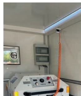
Image: Trailer with fixing system, socket strip and LED light rail
